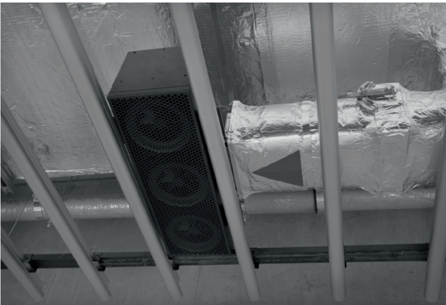
Fixed air pattern ceiling diffuser for mixing systems, size 675 x 188 x 225 mm. Airflow/unit 100l/s or 360 m 3 /s.
