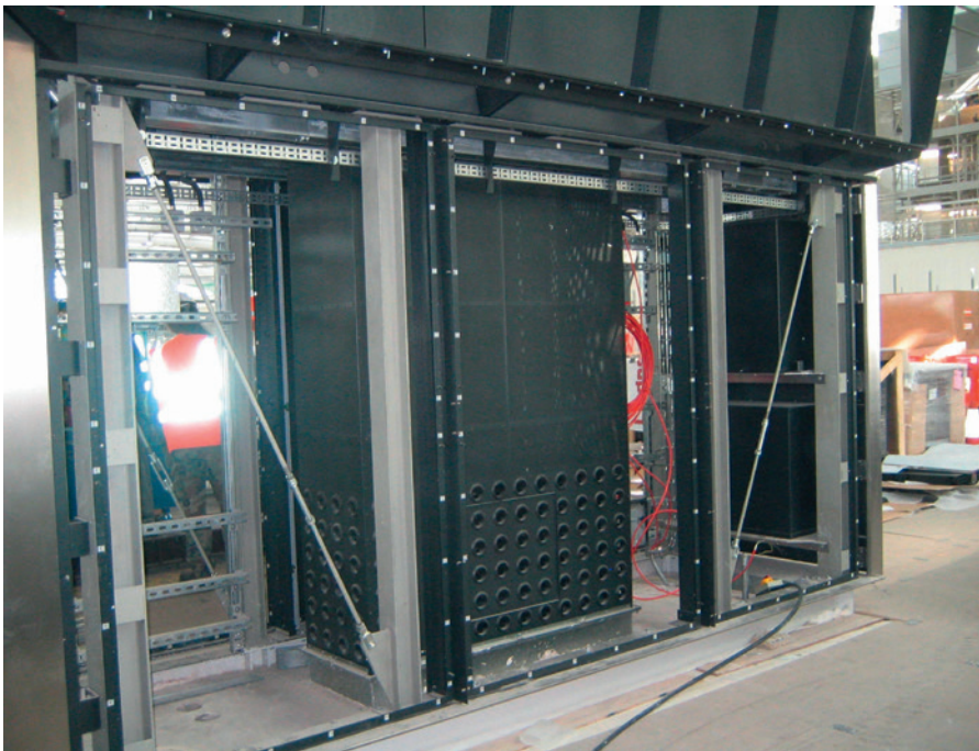
Diffuser steel frame construction with installed air distribution duct and fixing frames
