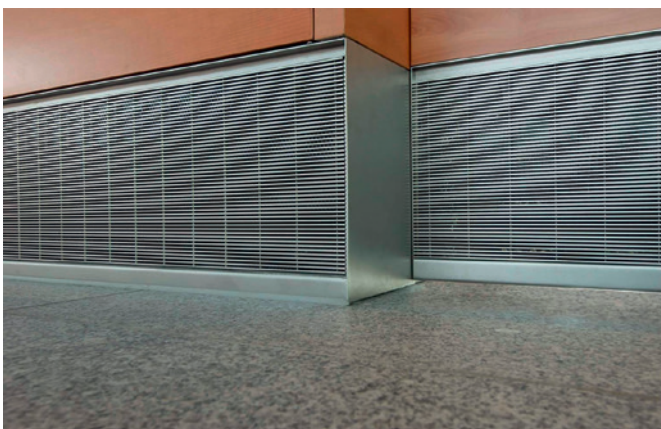
Plinth diffuser with stainless steel LSE grill. Supply air spigot from the back or from below.
