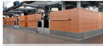
Stuttgart Airport, Terminal 3, Germany Plinth diffuser integrated in the front of counters. Front face built of shock proof stainless steel LSE material.
